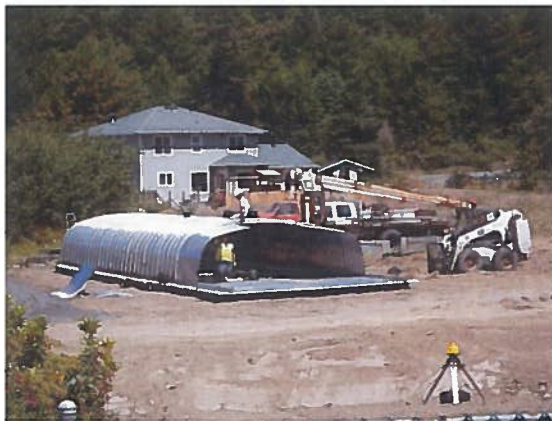
Assembly of arch culvert (Phase 1).
