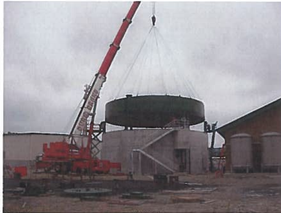
Installation of floating cover for anaerobic digester.
